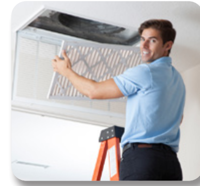
The higher the MERV rating, the more effective a filter will be in removing particles from indoor air.
