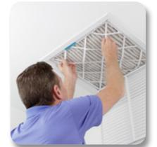
The higher the MERV rating, the more effective an air filter will be at removing particles from indoor air.
