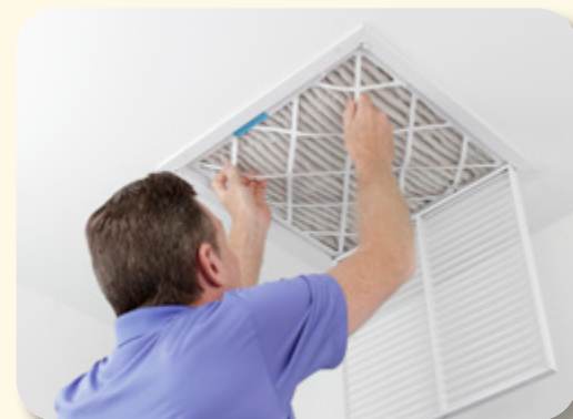
The higher the MERV rating, the more effective an air filter will be at removing particles from indoor air.
