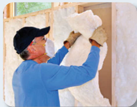
Proper insulation holds heat inside during the winter and keeps it from coming in during the summer.
