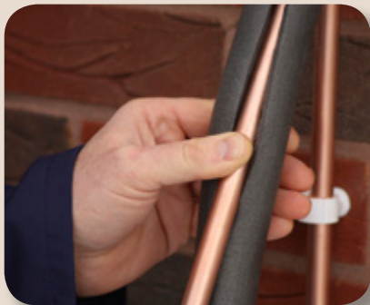
Foam insulation tubes can be an easy way to help protect pipes from freezing temperatures.
