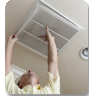
A clean air filter prevents dust and dirt from building up in your system. Buildup could lead to early system failure.
